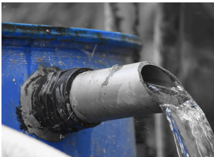
Water Desalination System, tzahiV de Getty images
